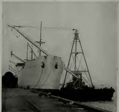
Photograph shows Smith-Rice derrick barge in Los Angeles harbor reaching over the MS Dagmar Salen and "picking" a lift from a gondola car. The ship's rail to water is 33 feet.
